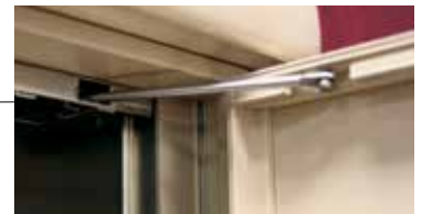
Stainless steel hold open door catch on each side of master gate
