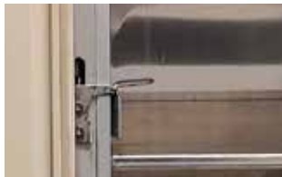
Easy release handle to open master gate
